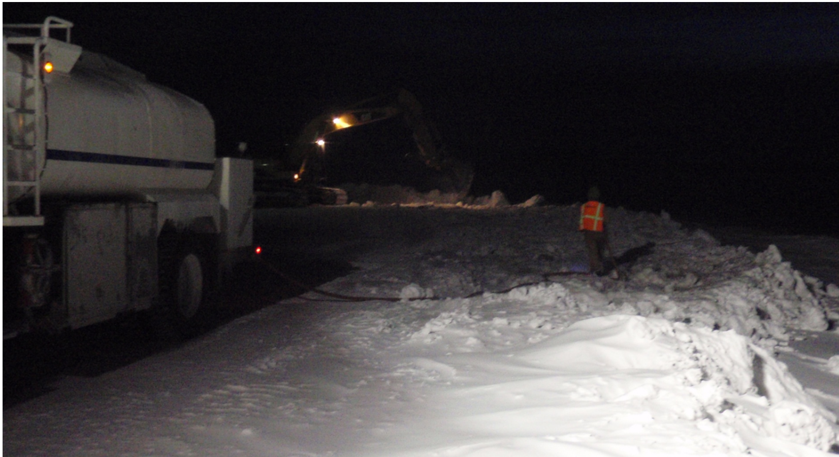
Photo 11: Snow being spread and watered near the west extents of the FCP Plant Pad.
