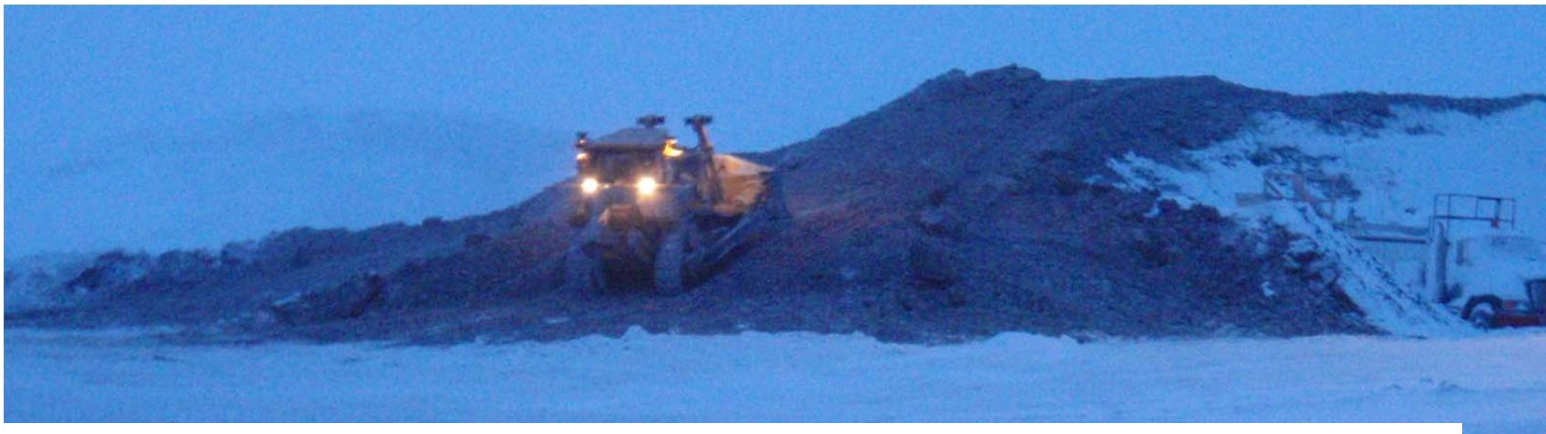
Photo 6 (above/ top right): Dozer working transition material stockpile by the Batch Plant (near Quarry #2)
