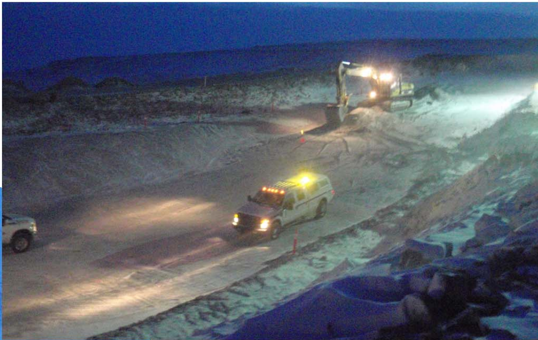
Photo 8 (center): View of excavator working on 5/8" material and survey checking grades in the central portion of the key trench.
