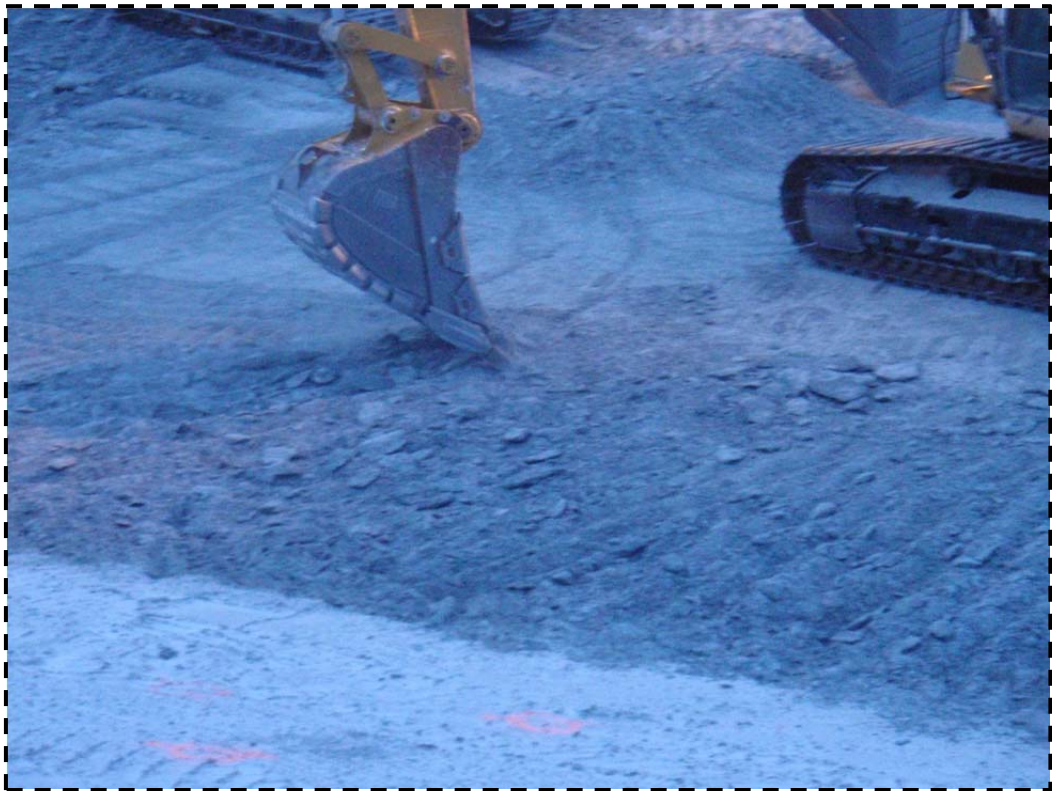
Photo 3 (bottom left): ~WNW view of the excavators removing frozen 5/8" material from the key trench.
