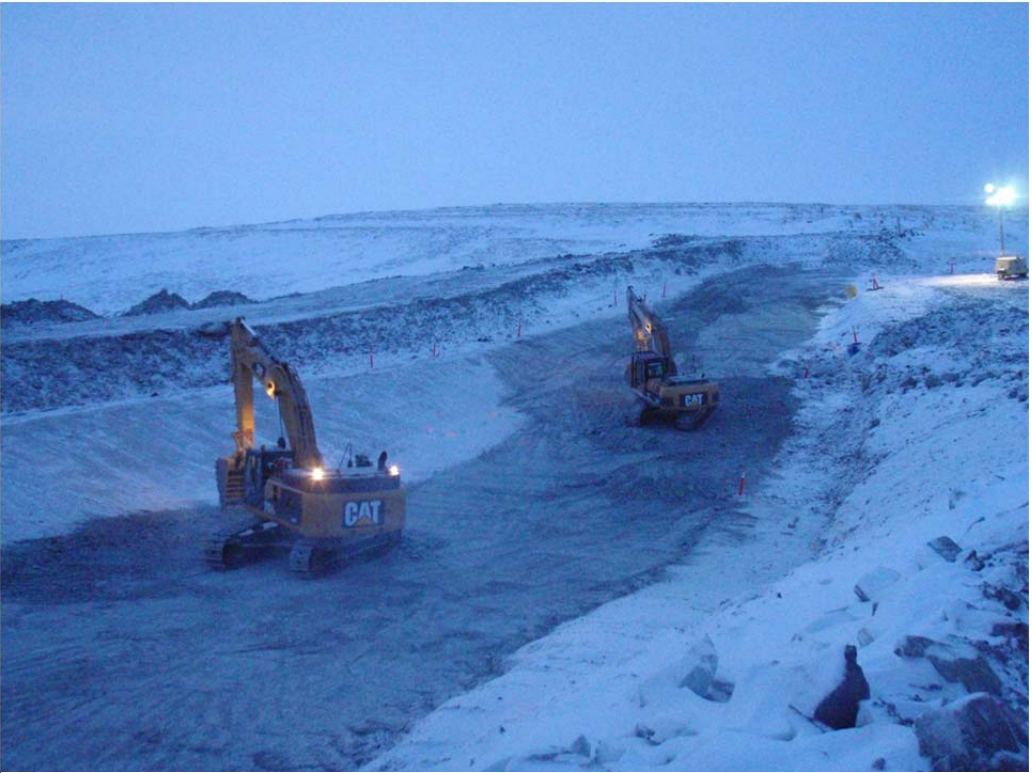
Photo 2: ~SW view of the excavators removing frozen 5/8" material from the key trench.
